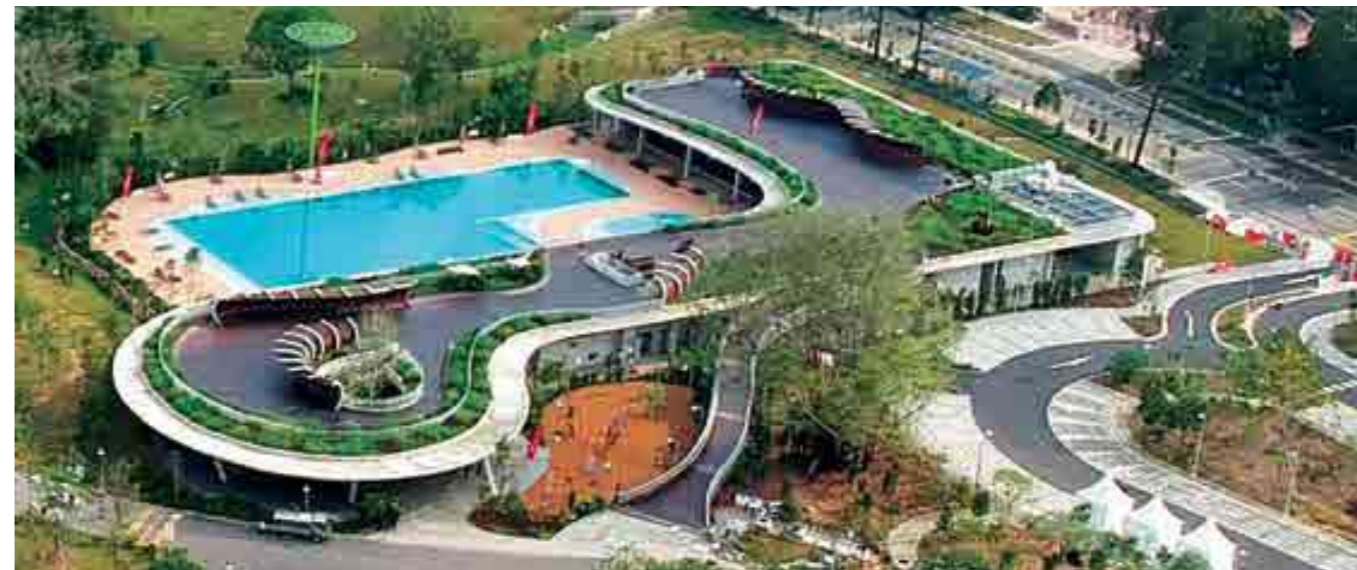
The site of the former Jurong Drive-in Cinema was first occupied by Fairway Country Club before it was demolished to build the ActiveSG Park as part of Jurong Lake Gardens. Courtesy of NParks.
